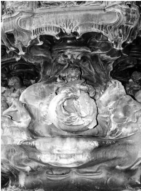
The Shaftesbury Memorial in London's Piccadilly Circus prior to conservation, left, illustrating the common problem of heavy limescale deposits on bronze fountains whose
